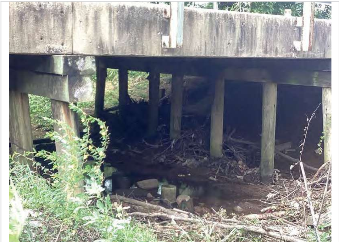
Bent 2 front side
