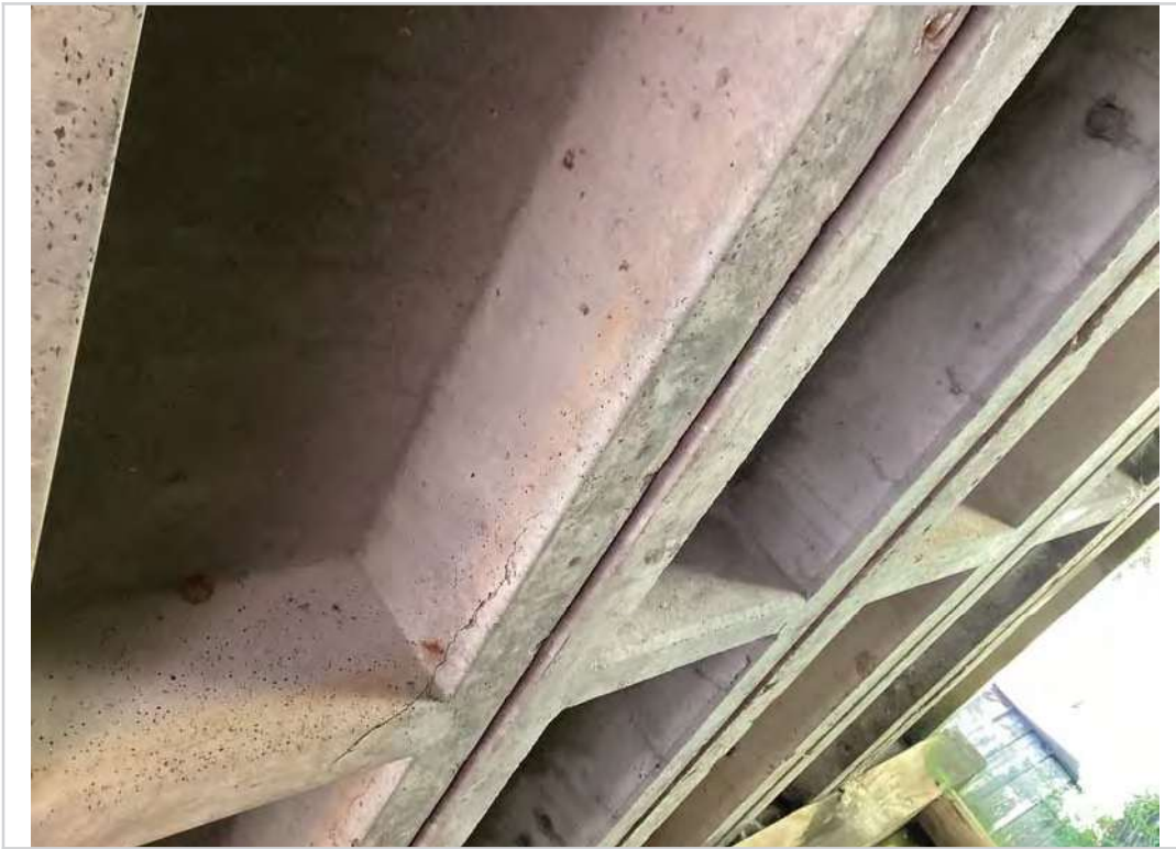
Span 1 bottom deck
