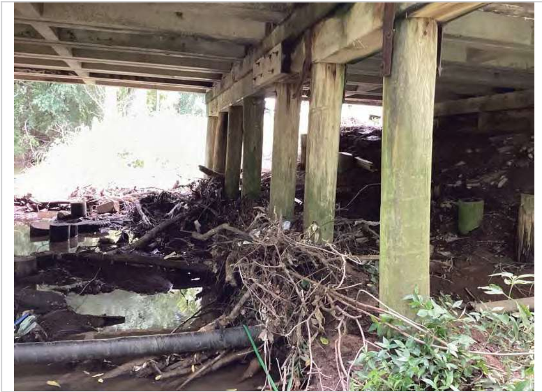
Bent 1 rear side
