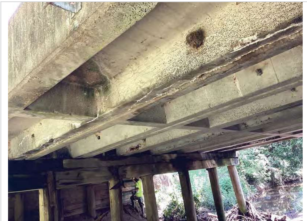
Span 2 bottom deck
