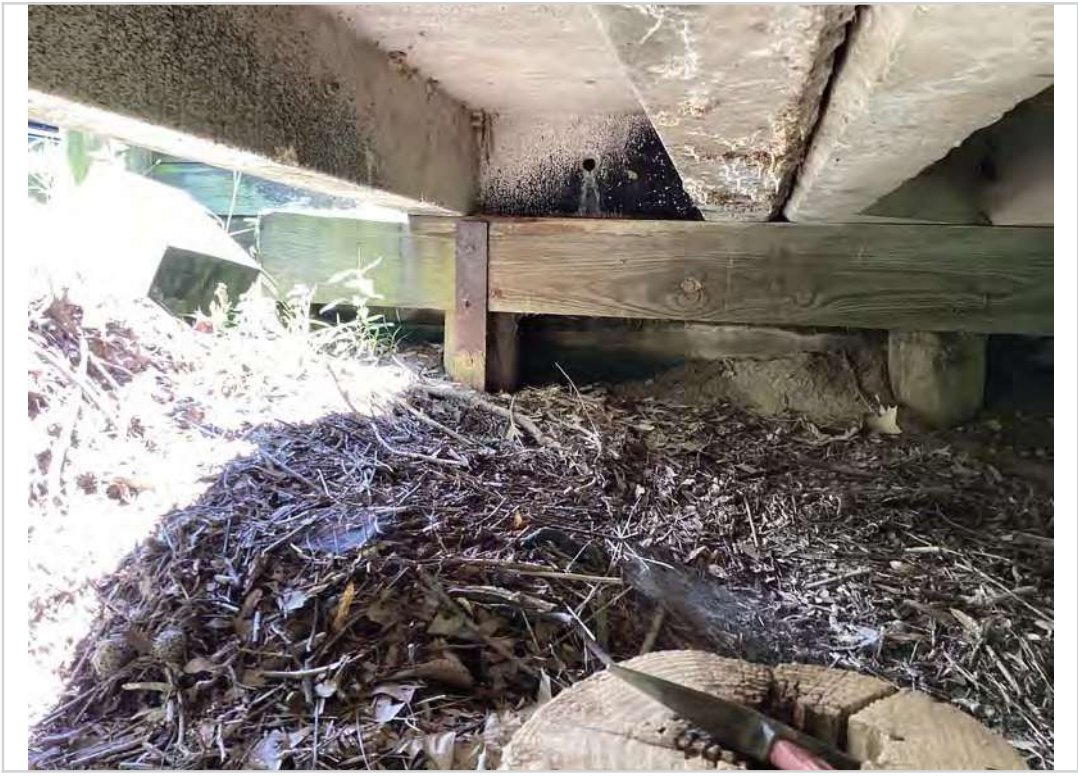
Abutment 1 pile G
