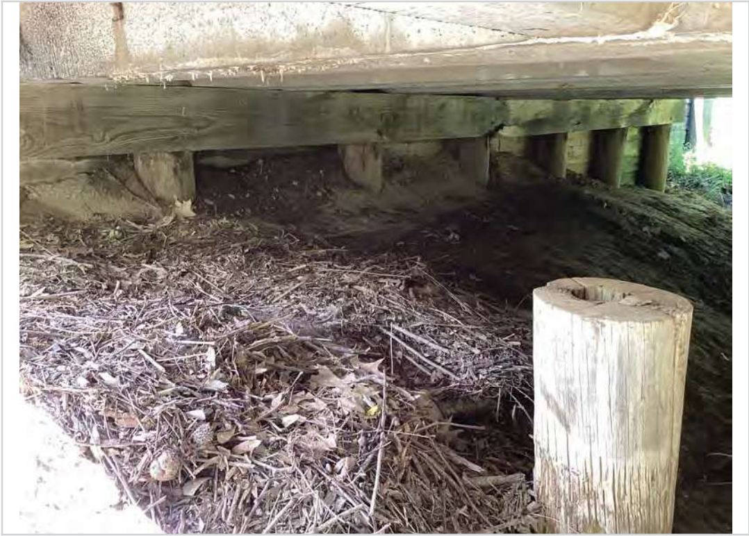
Abutment 1 looking back
